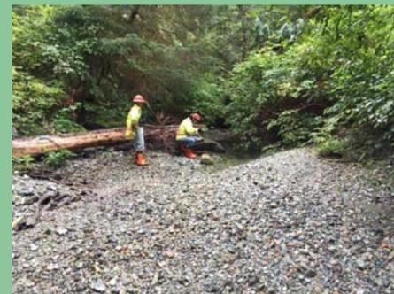
These photos show a side channel of a stream restoration project (see good practice in the text at left). The large boulders on the top photo and logs on the lower photo were installed based on a biologist’s recommendation to create pools which were previously absent. The person in the lower photo is observing fish in a small pool at the end of the dry summer season, demonstrating the habitat enhancement was successful.
