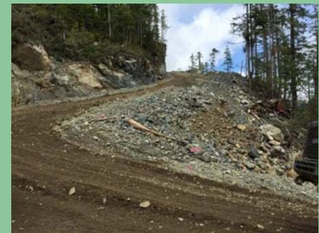
The road shown above was confirmed to have been constructed in accordance with the prescription developed by a terrain stability specialist to manage risk of slope failure. This section of road is at 26% grade and accesses a hanging valley with several cutblocks which were also assessed during the audit.
